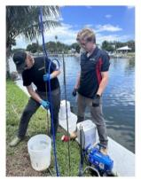
In June of 2024 permeation grouting of a single component polyurethane foam, HS010, was conducted between the depths of 3 to 10 feet below grade. Spacings of the injections were approximately 2 feet on-center. A pre-determined amount of HS010 (between 9 and 14 lbs) was injected every foot.
